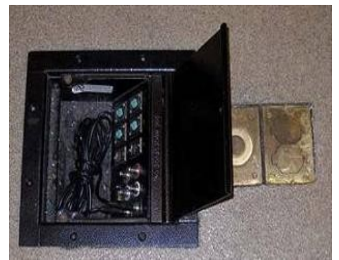
Theatrical Box In Center Of Hall With XLR Microphone, Audio & Video Hookups Plus 110V and 220V power. Example: a lighted table and fountain can be placed in the mid-
